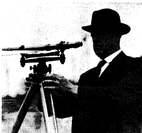
Frederick M. Smith, At the Auditorium Construction Site, 1926
