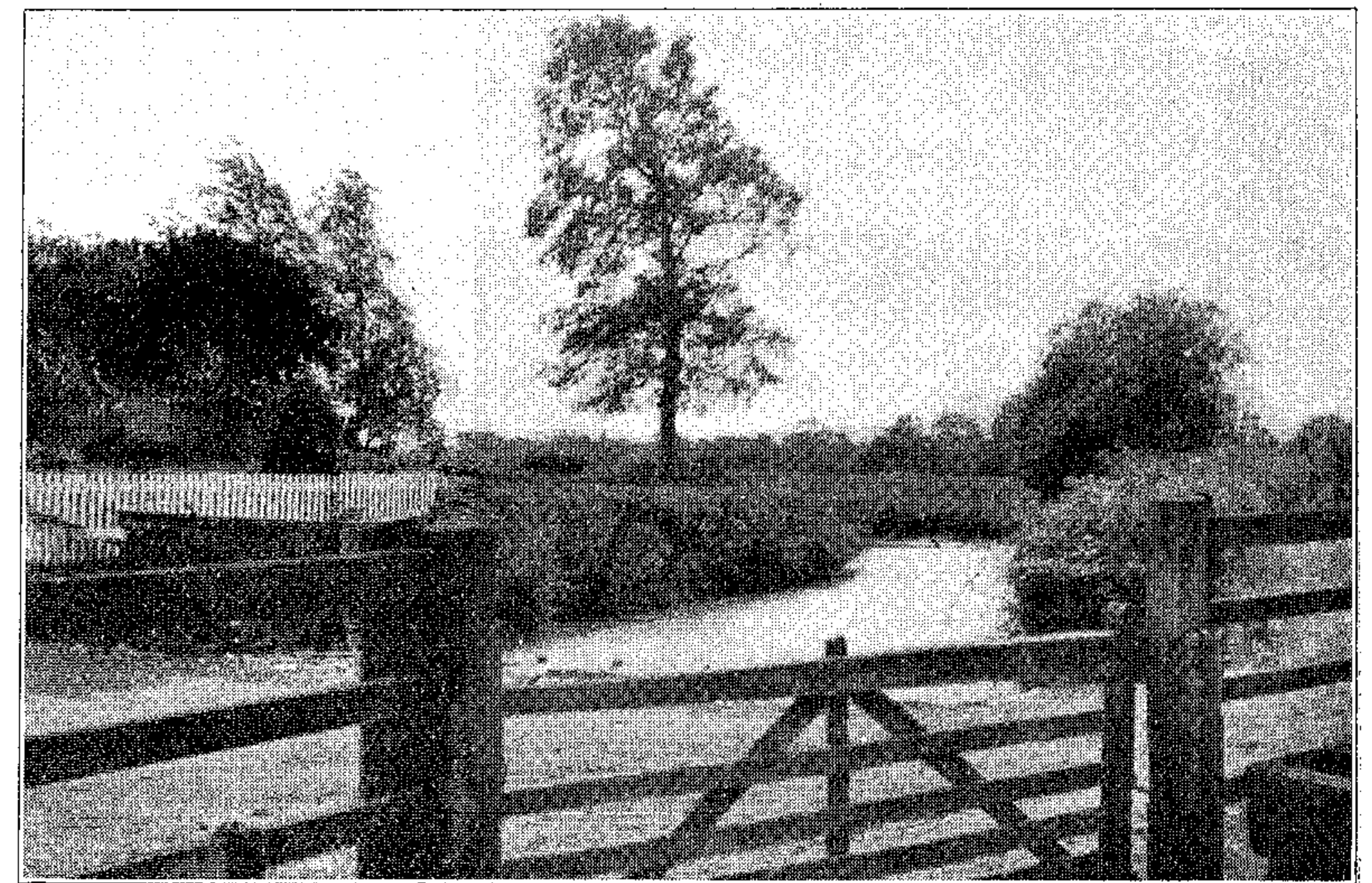
Picture taken in 1912 showing the moat about Olmsted Hall, Essex, England, with the section where the ancient drawbridge was located having been filled to make a roadway to the barns.
